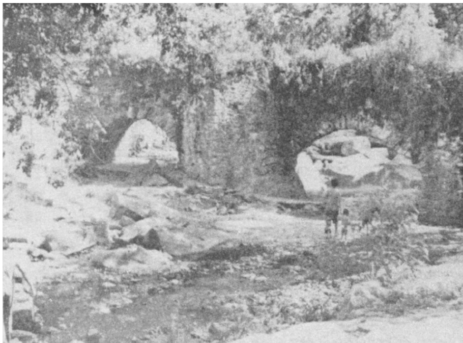
b. Espada Aqueduct in 1977
