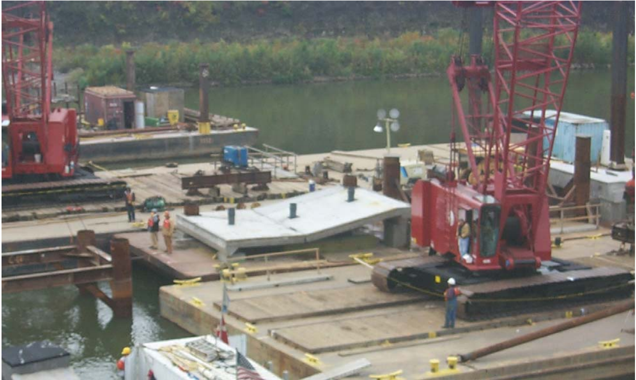
Figure C-14. In-the-wet tailrace panel installation for Braddock Dam
