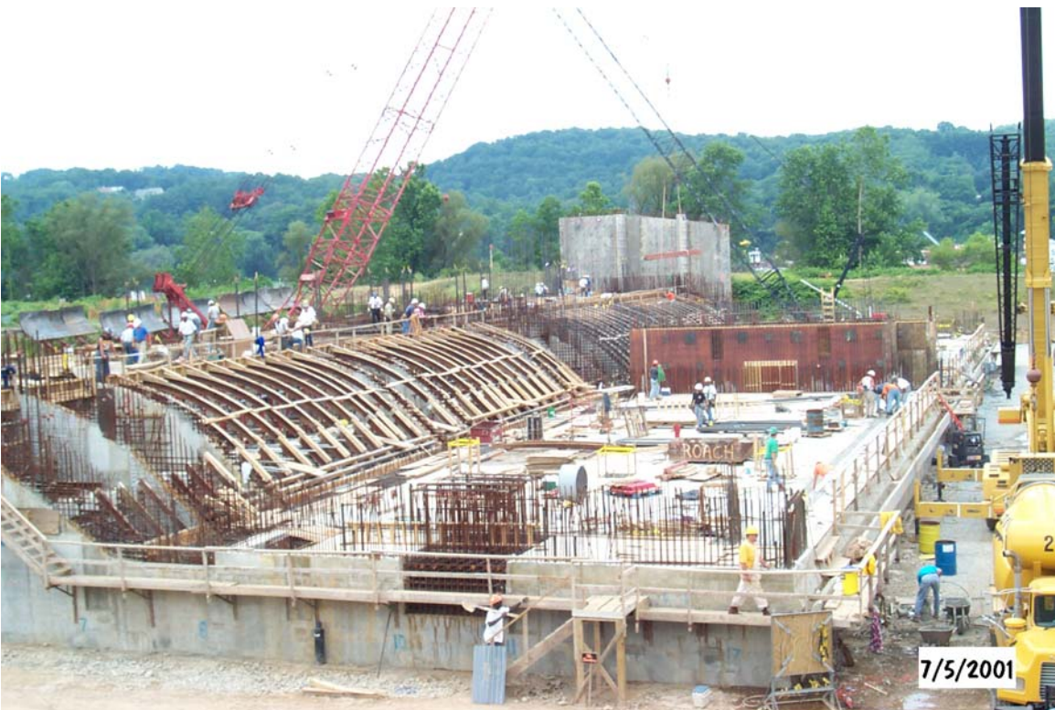
b. Construction of dam Segment 2 within the two-level casting basin Figure C-11. Assembly of float-in Braddock Dam at casting facility
