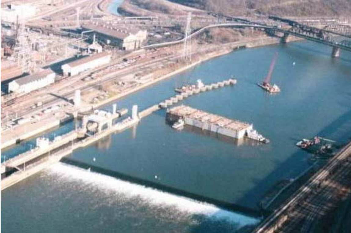
a. Initial positioning of dam Segment 1
