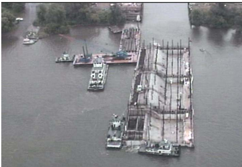
b. Float-out or launch of the first segment of the dam Figure C-10. Braddock Dam Casting Facility
