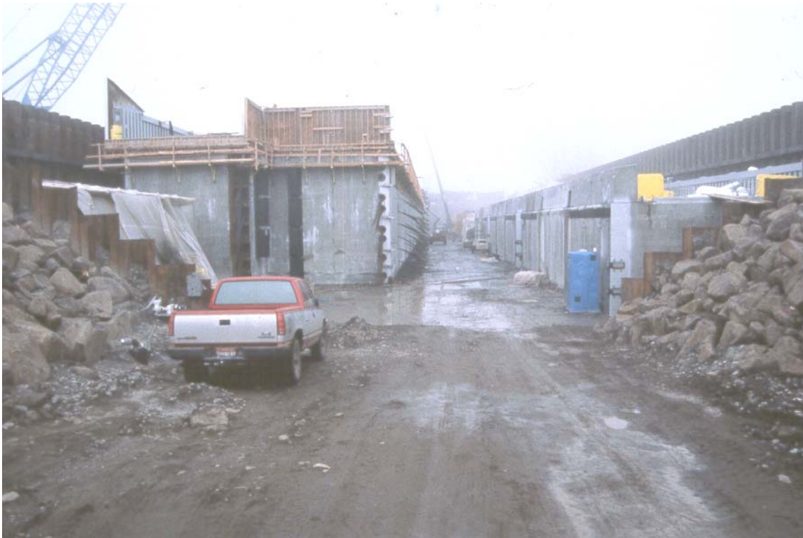
Figure C-21. Precast yard in Bordman, Oregon, for Bonneville Project. The contractor constructed a graving dock. The pontoons were fabricated, the site was flooded, and the pontoons were towed to Bonneville for installation
