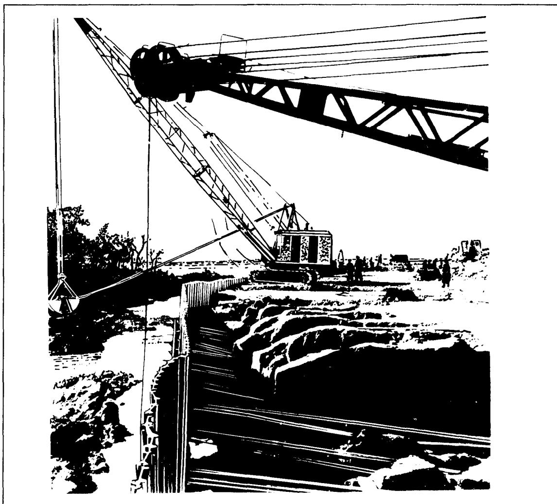
Figure 7-1. Bulkhead Using Steel Sheet Piles and Tie-Rods
