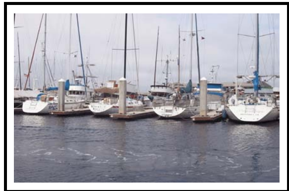
Fingerfloat Piles Adjacent to Channel
