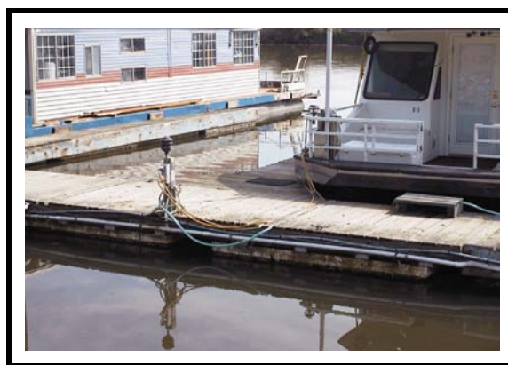
Utility Lines in Walkway Deck Gaps
