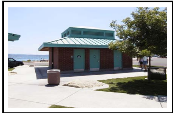
Unisex Toilet Compartment Restroom
