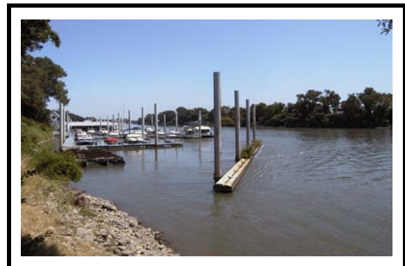
Upstream Debris Deflection Boom
