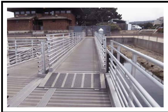
Handrails on Both Sides of a Gangway
