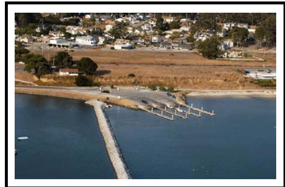
Boat Launching Facility Within Marina Basin
