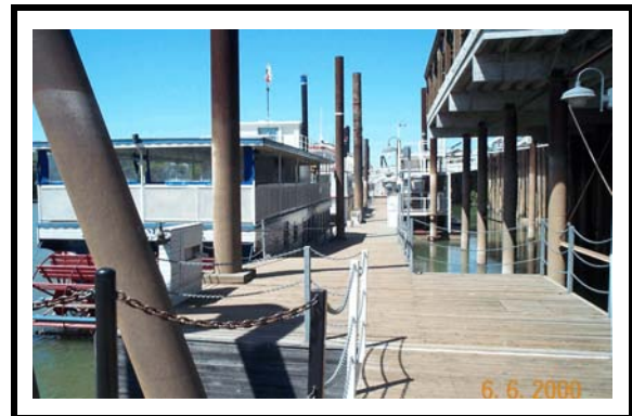
Steel Guide Piles in a River Marina
