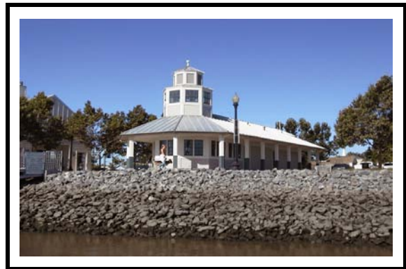
Marina Restroom Facility
