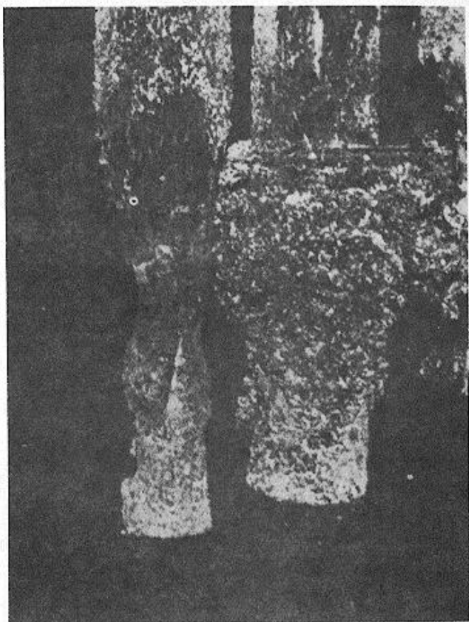
Figure 2-2. Destruction of wooden piers by marine borers.
