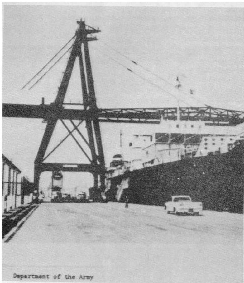
Figure 12-3. Typical rail-mounted gantry crane.
