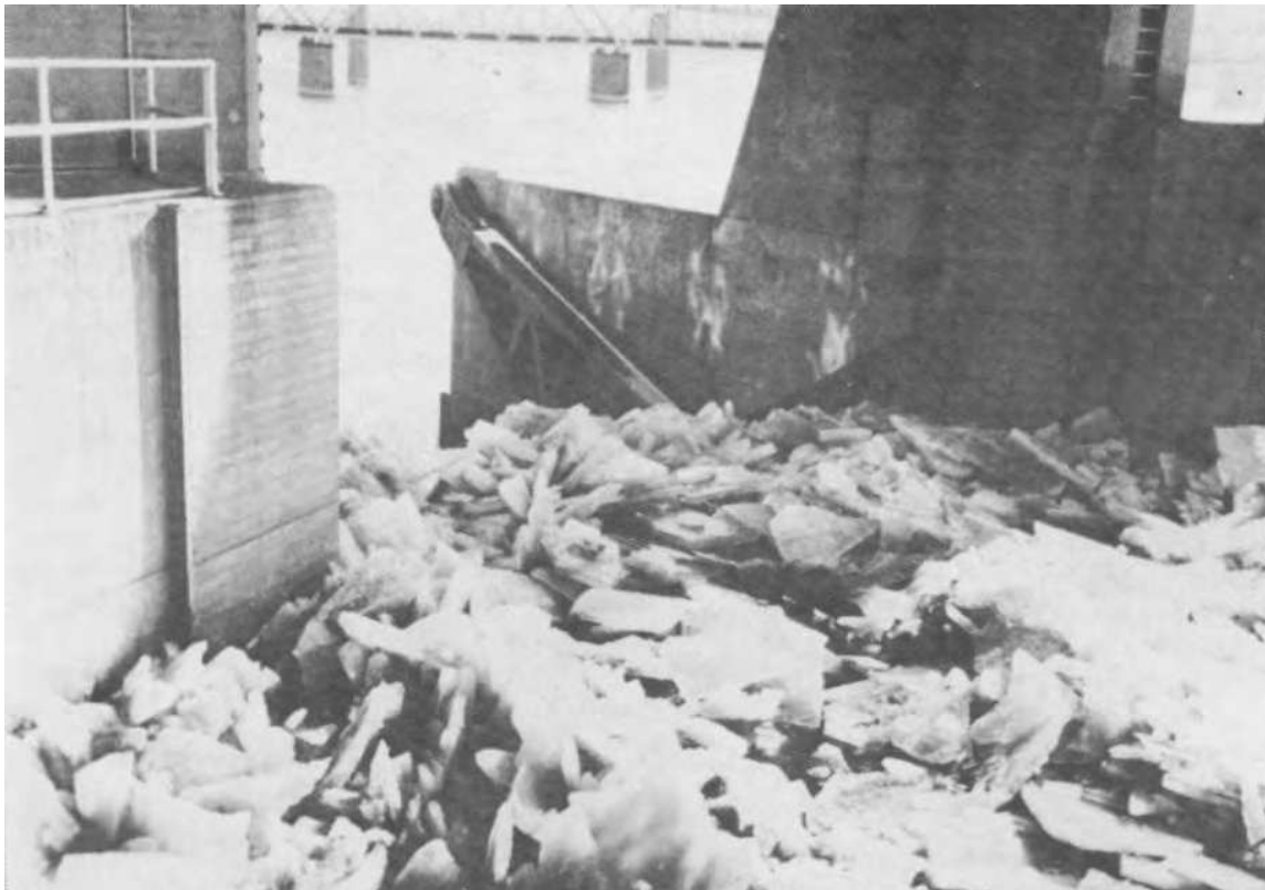
Figure 5-23. Ice on control gate
