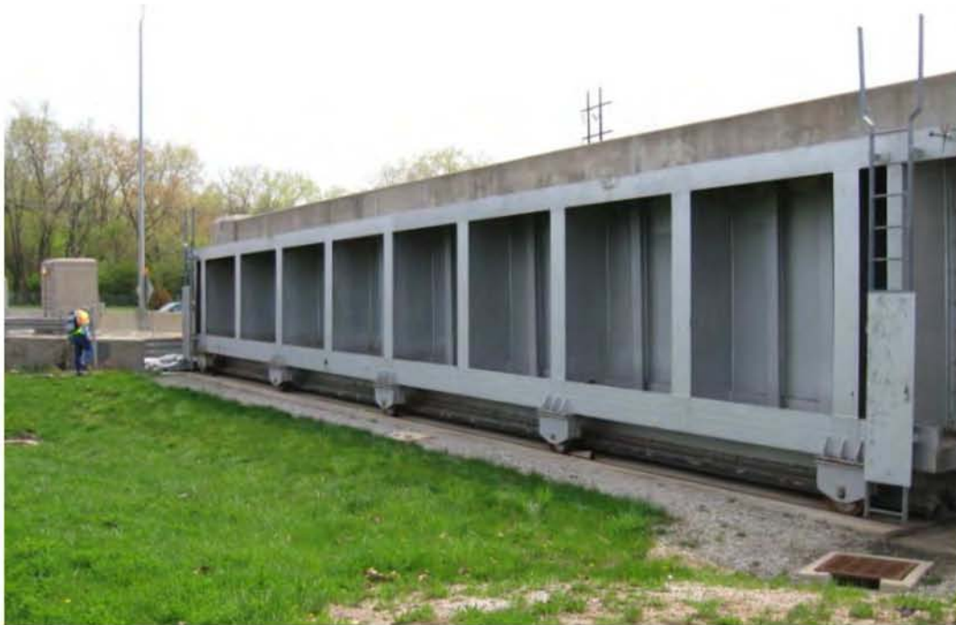
Figure F-5. Rolling Gate Closure Structure.
