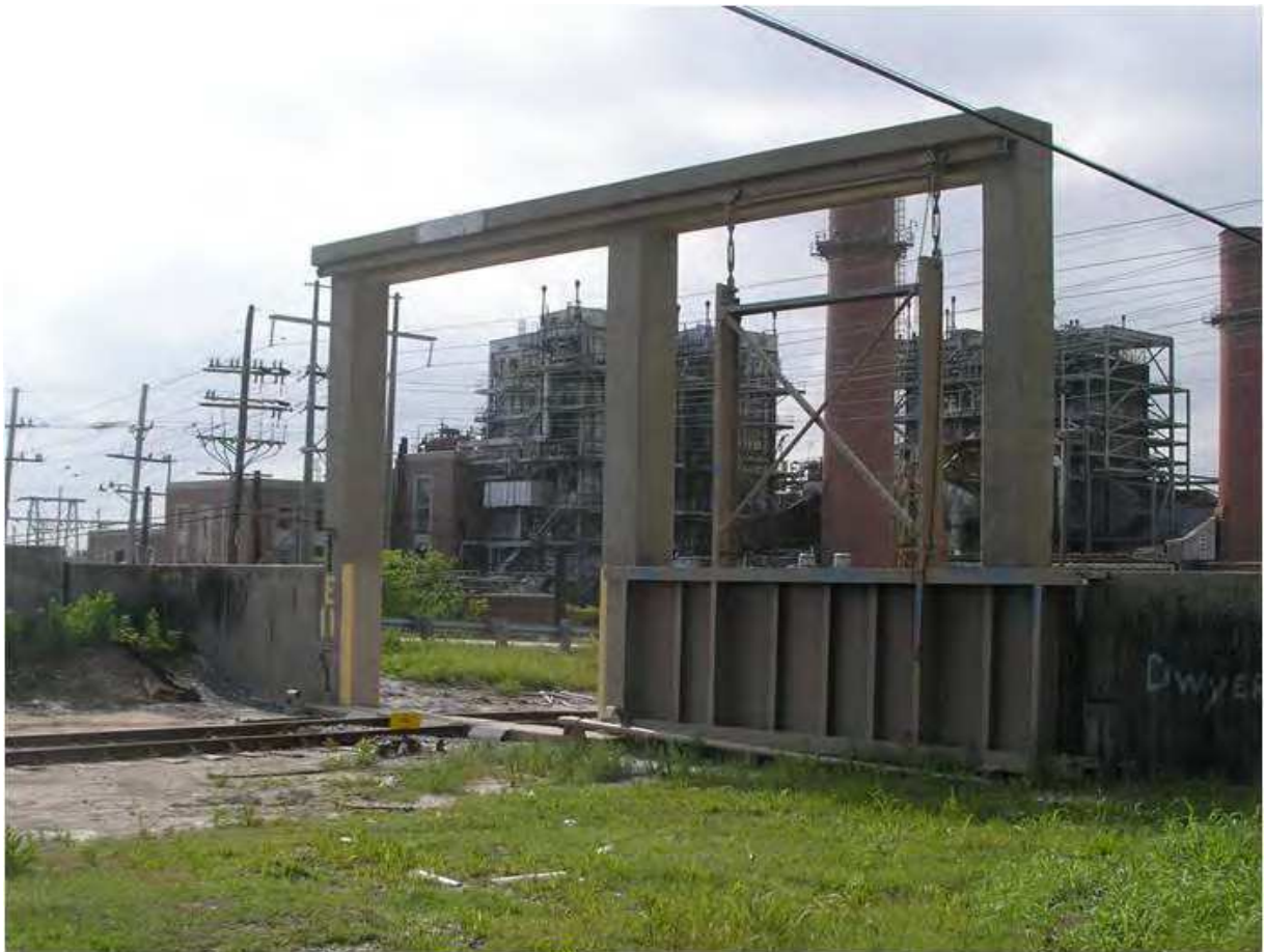
Figure F-7. Trolley Gate Closure Structure.
