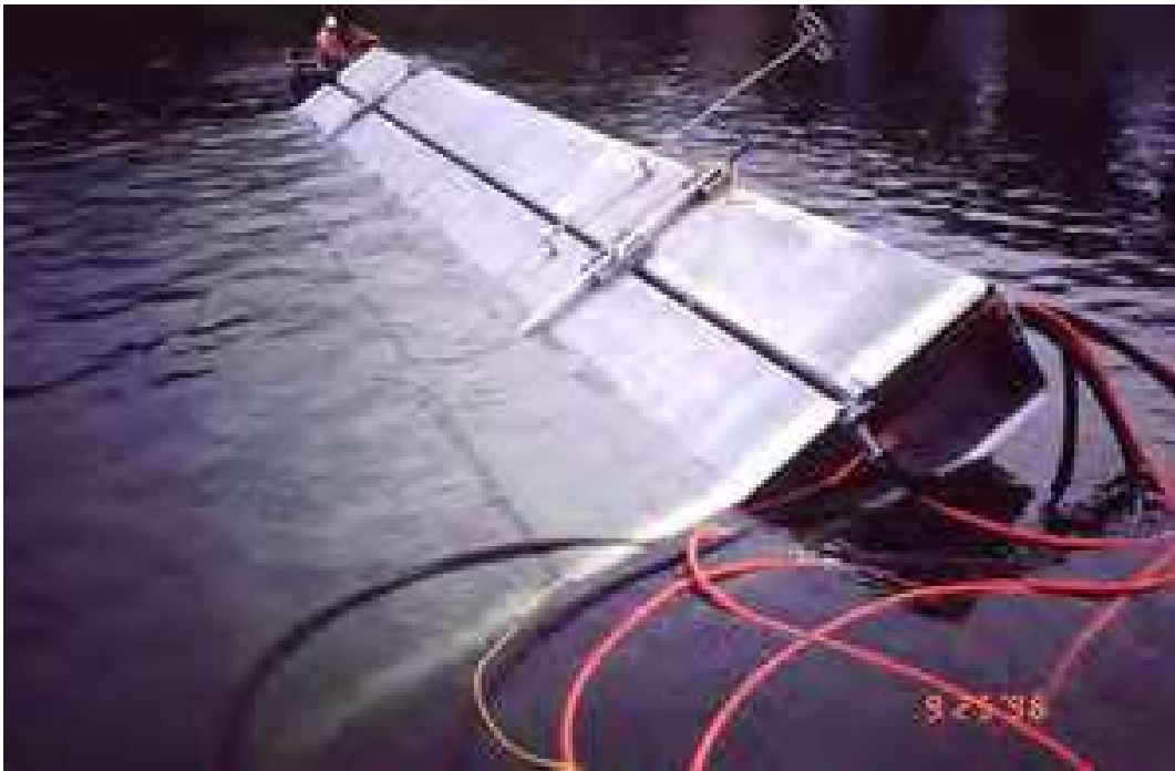
Figure B-9. Floating Bulkhead.
