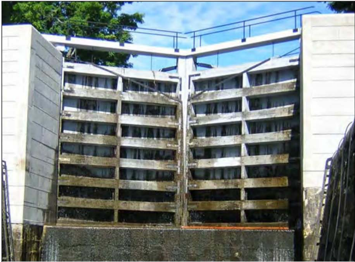
Figure B-1. Miter Gate.
