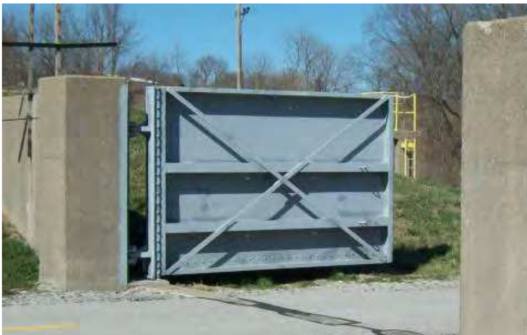
Figure F-2. Swing-Gate Closure Structure.
