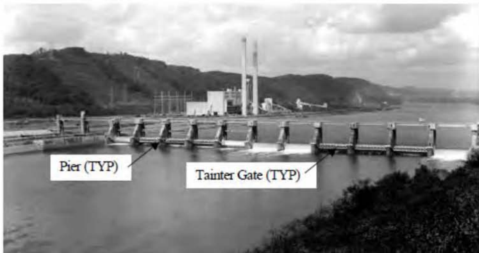
Figure D-1. Overall View of Navigation Dam from Downstream.
