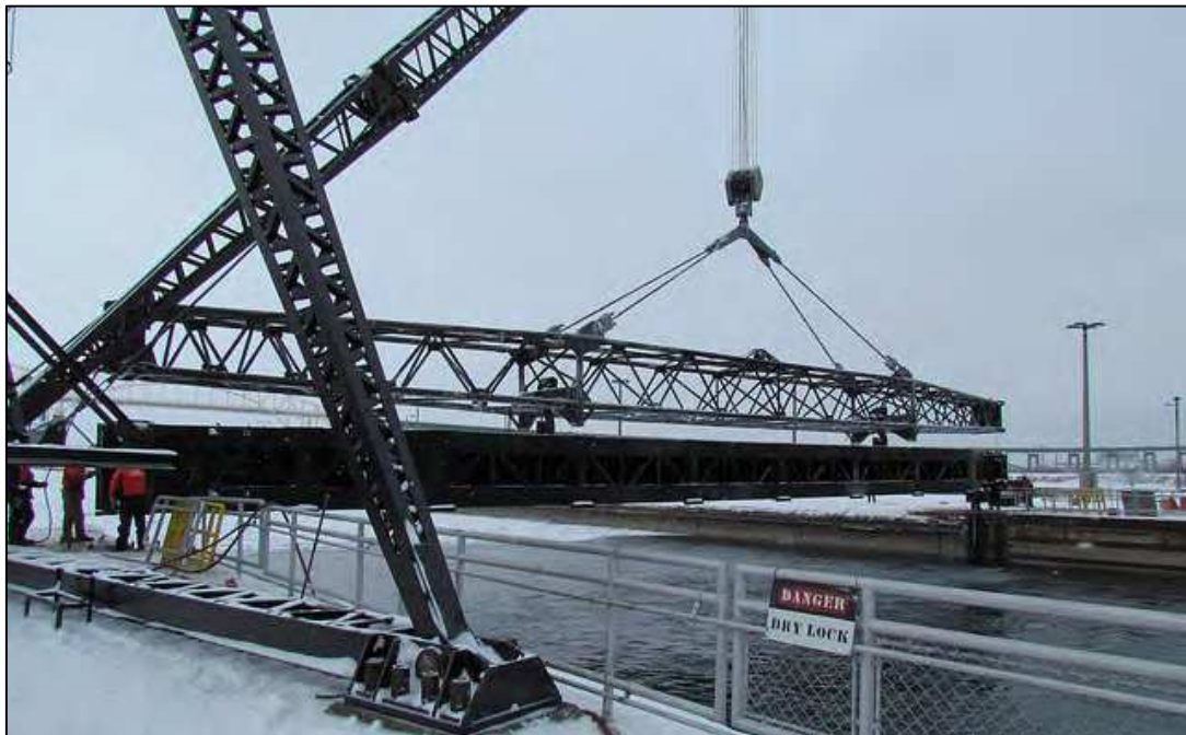
Figure B-10. Lifting Beam.
