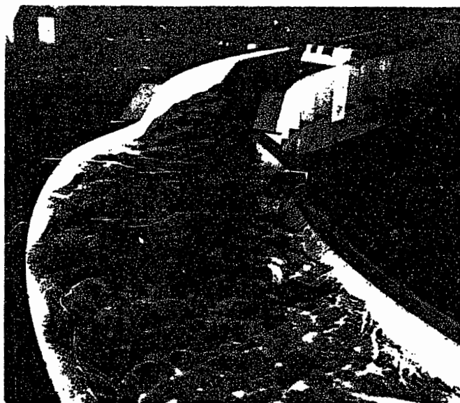
Without suppressor - waves overtop canal.
