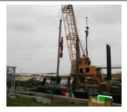
Figure 12-4 Hoisting Hammer and Lead
