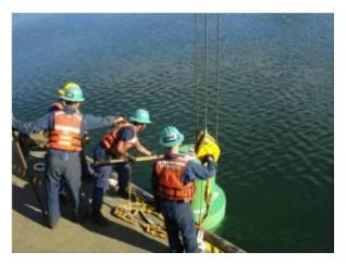
Figure 10-1 Hooking into the Buoy
