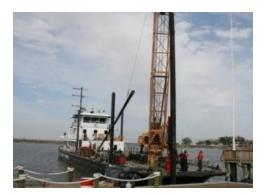
Figure 12-5 Crane Hoisting Pile
