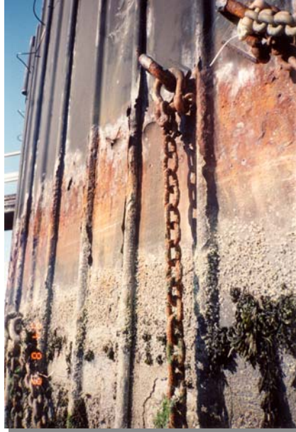
Photo 3-7 - Coating Deterioration in the Splash Zone
