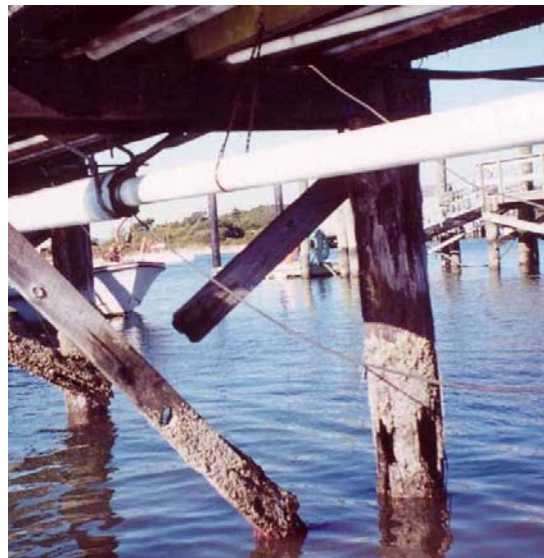
Photo 2-2 - Marine Borer Deterioration of Bracing and Pile in the Tidal Zone
