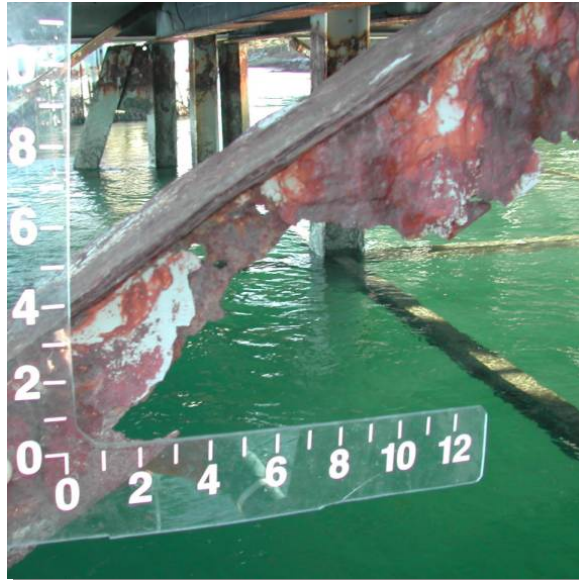
Photo 3-3 - Severely Deteriorated Wale (Note knife edge flange)
