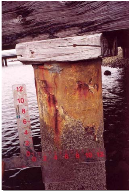
Photo 4-1 - Rust Staining of Concrete Pile
