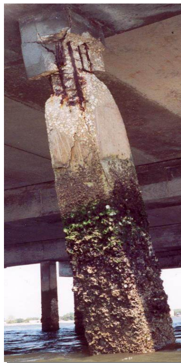
Photo 4-4 - Failed Repair with Exposed and Corroded Reinforcing
