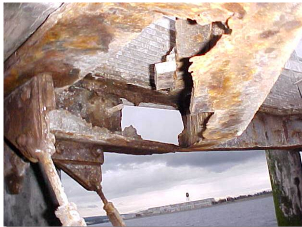
Photo 3-4 - Severely Corroded Steel Framing
