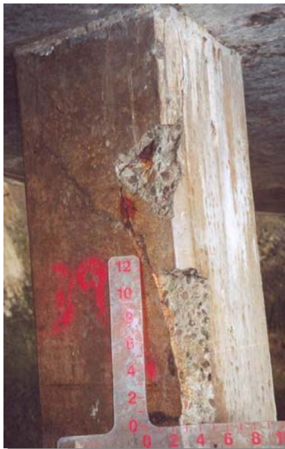
Photo 4-2 - Vertical Crack and Spall
