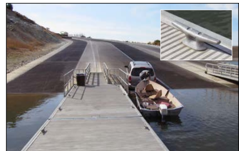
minimum of 5 ft clear between edge hardware
