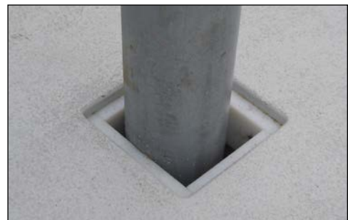
square pile yoke with rub strips
