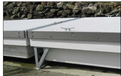
support leg adjacent to float hinge
