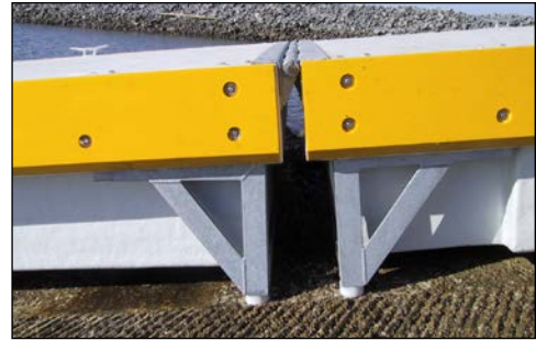
unnneeded downslope support leg(s)
