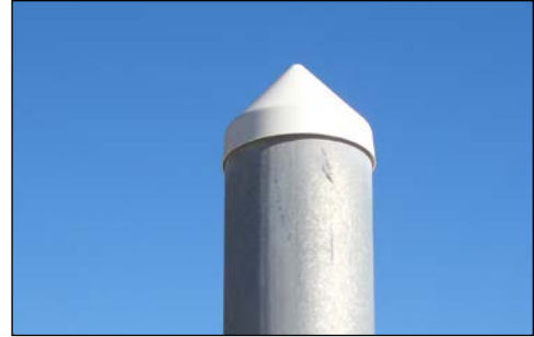
guide pile with "cone" cap
