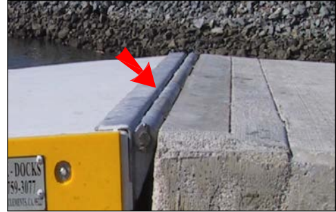
boarding float-abutment hinge
