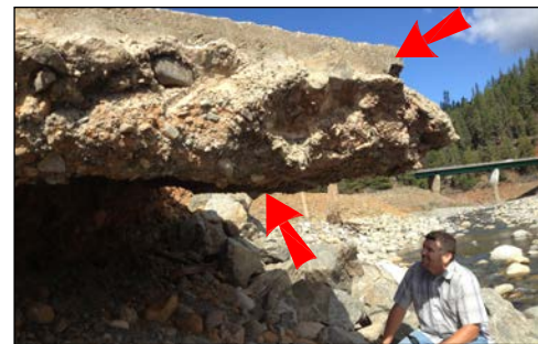
flood water undercut launching ramp
