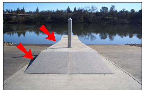
matching width of gangplank and float
