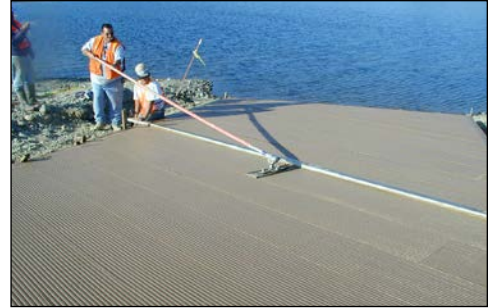
creating diagonal V-grooves in wet concrete
