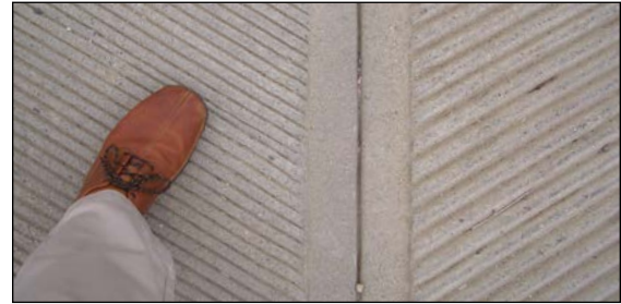
two-lane launching ramp 1 inch V-grooves on right lane 1/2 inch V-grooves on left lane
