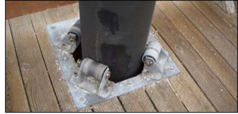
pile rollers wearing against round pile
