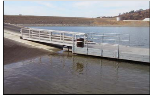
gangplank access to boarding floats
