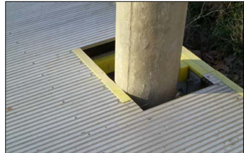
interior pile yoke flush with deck
