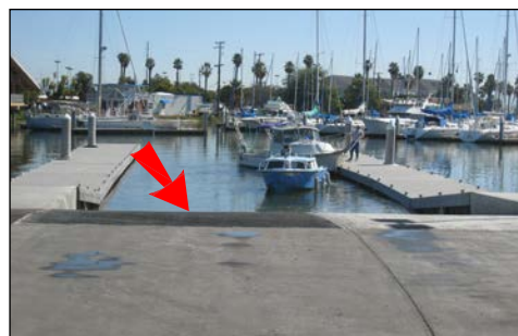
vertical curve at head-of-ramp
