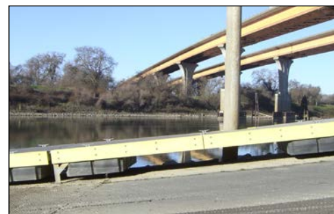
30 inch max. boarding float height
