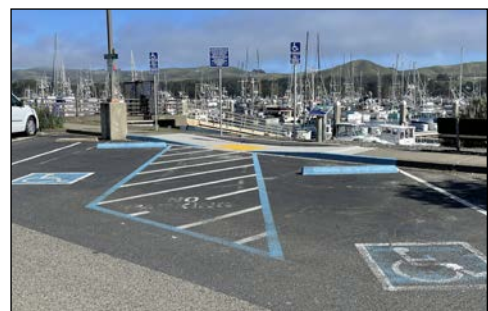
accessible ramp and access aisle
