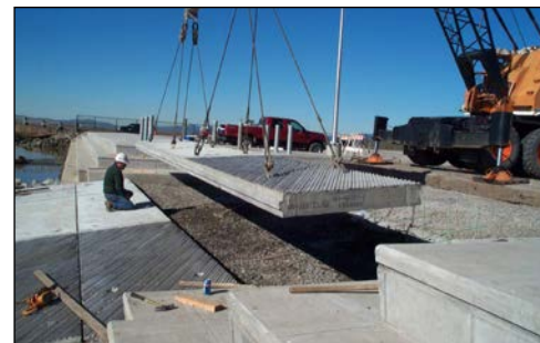
large precast concrete panels being placed
