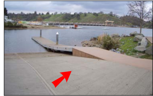
launching ramp apron merging with vertical curve
