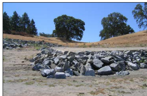
rock rip rap failing at bottom of a lake based boat launching ramp
