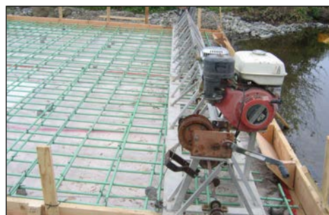
gasoline powered vibratory screed
