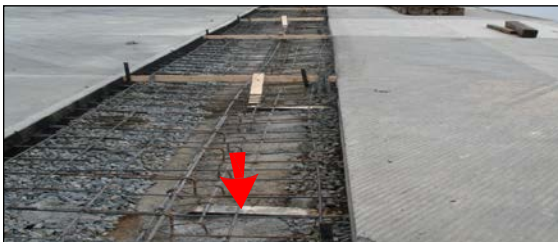
closure section under construction
