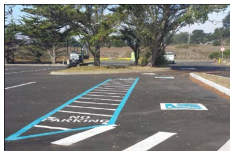
45 degree diagonal lines on 3 ft centers plus “NO PARKING” notification
