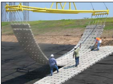
flexible cellular concrete mat
