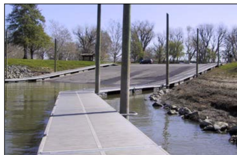
external guide piles along outside edge of floats
